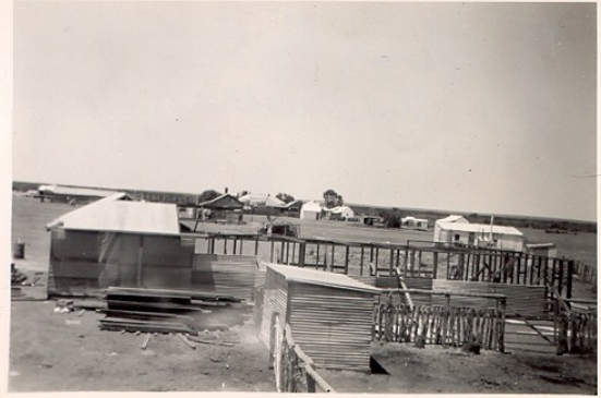
Building the new stables, 1950's.
